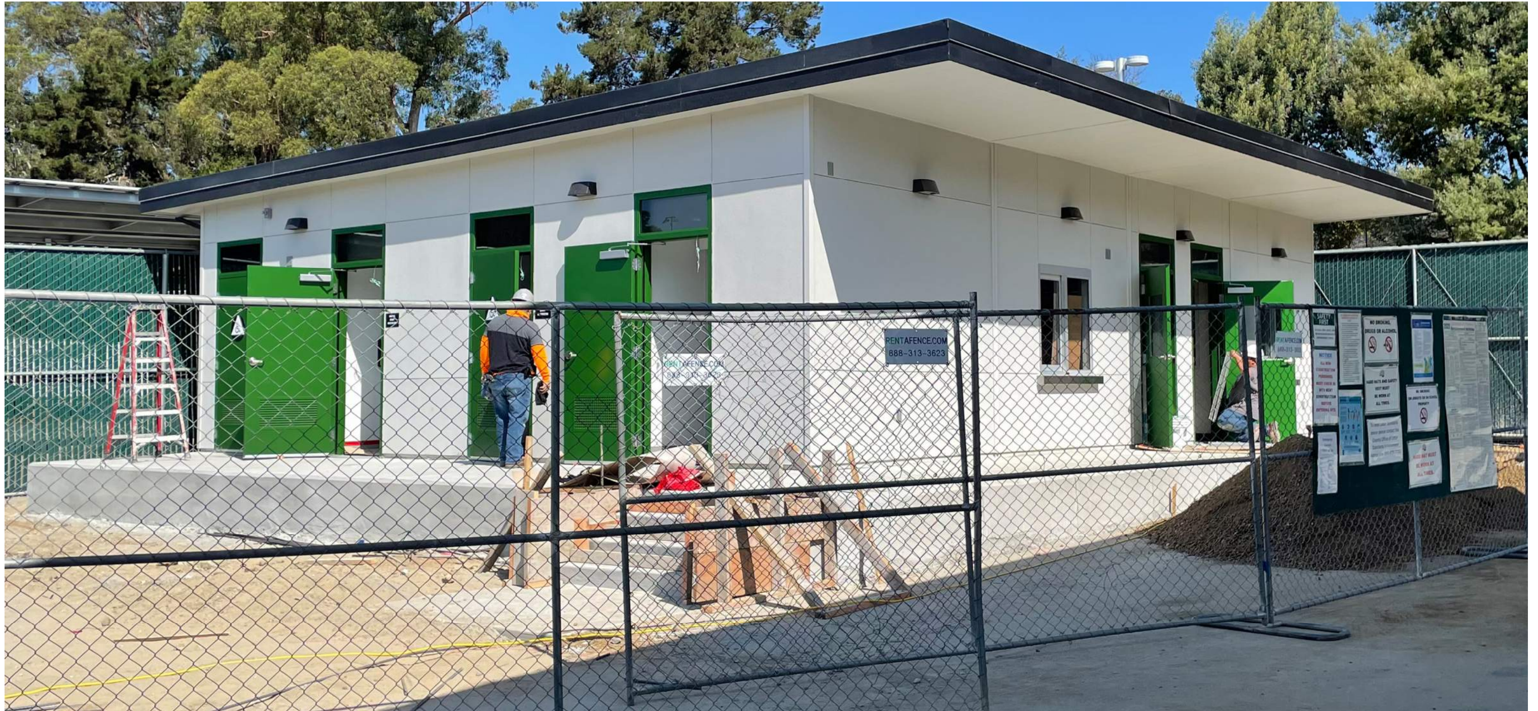
UNDER CONSTRUCTION – NEW TRANSPORTATION YARD OFFICE
